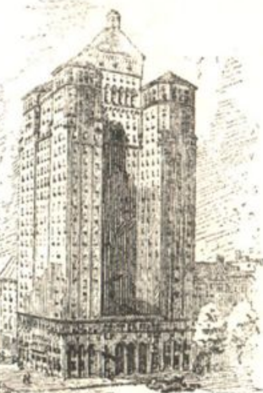
Huron Street & Michigan Avenue Chicago (Under Construction)
