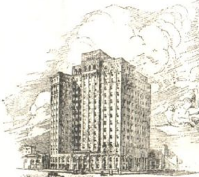
Chester Ave & East 15th Street Cleveland (Under Construction)
